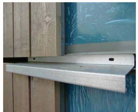
Metal flashing between each storey prevents the spread of fire.
