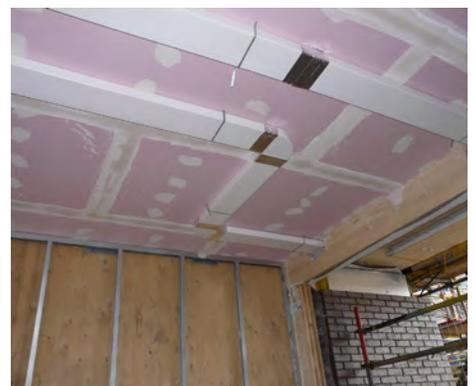
Building systems are routed through a ceiling void created with gypsum board.
