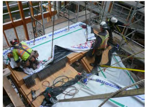
The 'free-floating' staircase connection to the landing using the Holz-Stahl-Komposit-Systeme (HSK-System)™. This system uses glue to connect the steel members to the wood.
