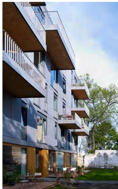
Exposed timber on underside of balconies at 3XGRÜN
