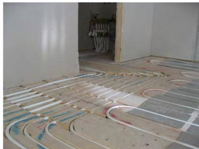
On-site milling for hydronic heating pipes at Limnologen
