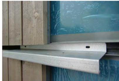
Holz8 exterior wood façade with metal flashing between each storey prevents the spread of fire
