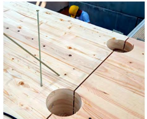
Cross screw technique used to connect floor and wall panels.
