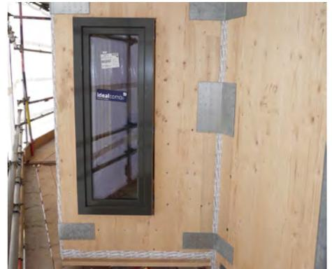
CLT floor panels and walls secured with custom gang nail steel plates.
