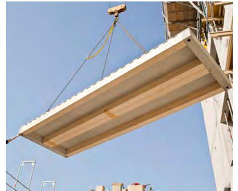
Hybrid floor slab features wood-concrete composite rib construction.
