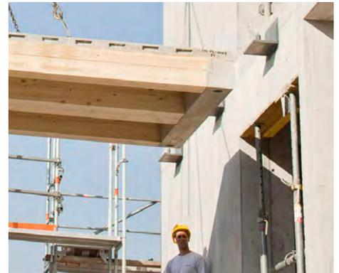
Angled steel brackets connect hybrid floor slabs to concrete access core.
