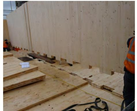
Interlocking keyed edge of each floor and wall panel.
