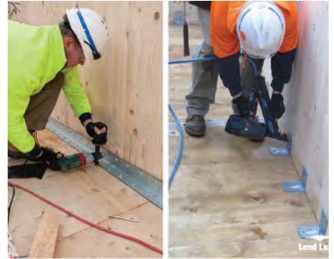
Angled steel connection plates and screws.
