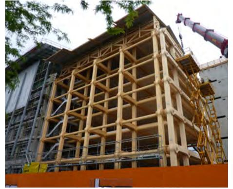
Temporary roof over timber structure
