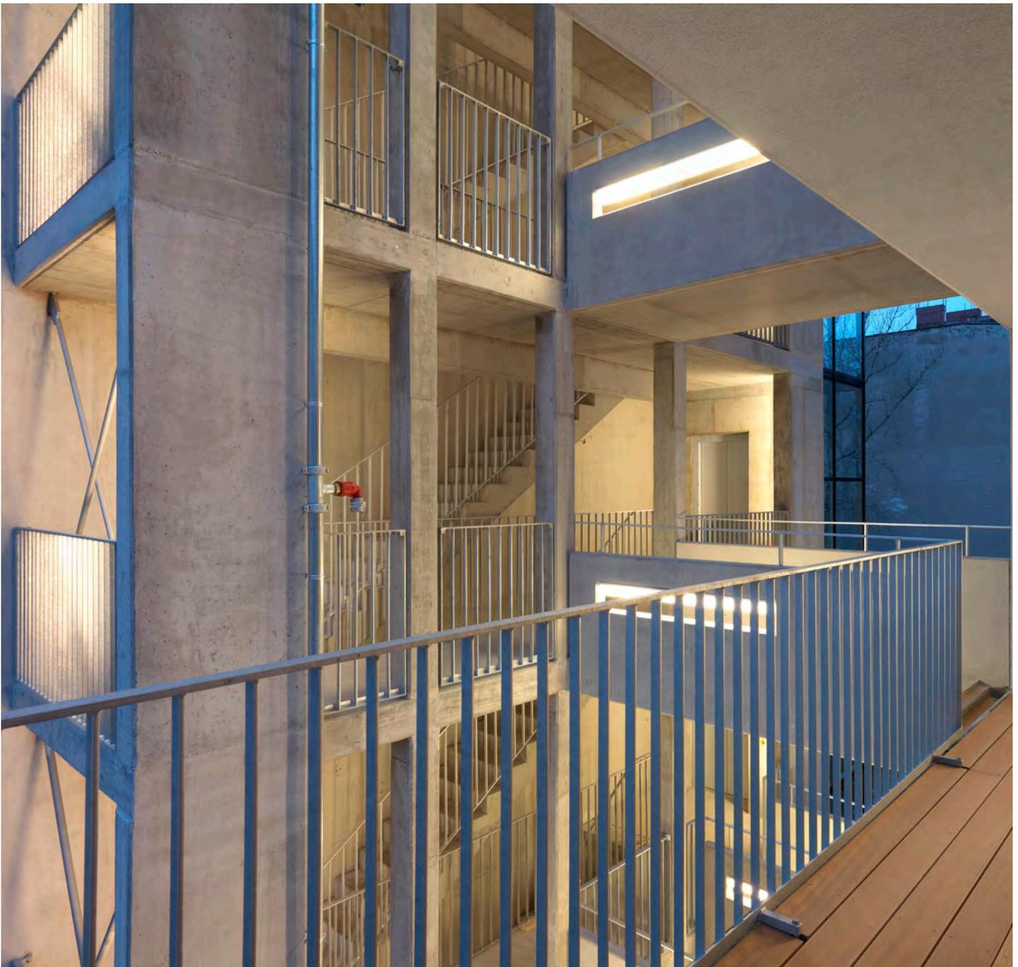
Exterior concrete stair and elevator shaft.
