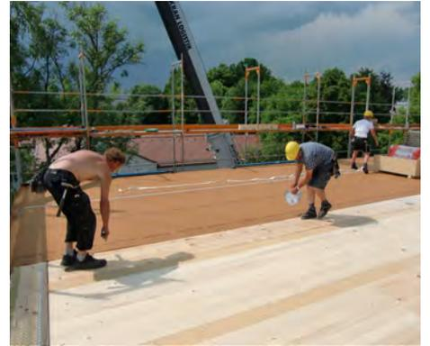
Floor panels covered with waterproof membrane after installation.
