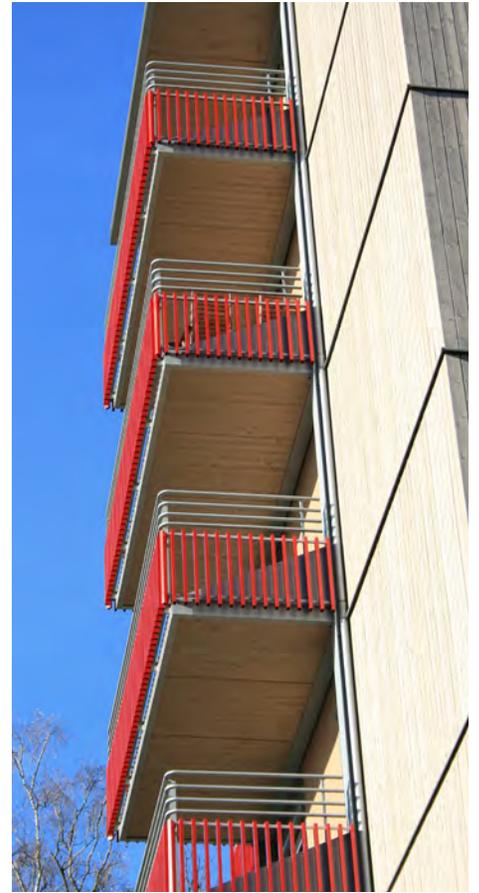
Timber balcony panels enclosed by steel frame
