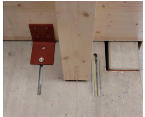
Steel bracket used to connect wood floor panels to concrete core.
