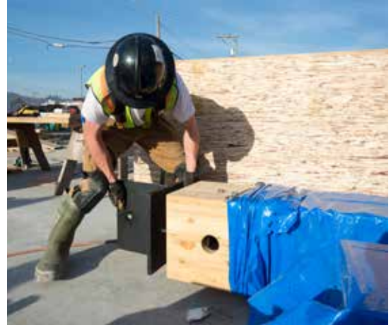
Glulam beam with steel connector Photo Credit: Paul Alberts
