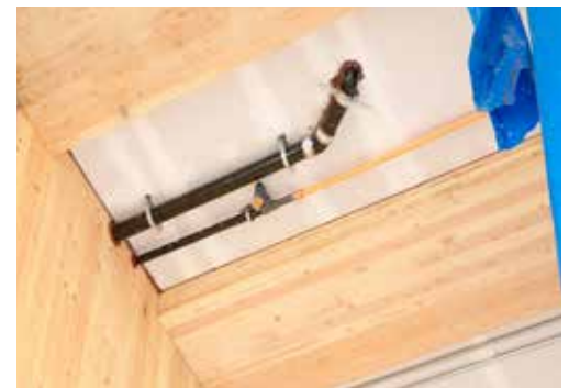
Services in chases, with penetrations through fire-rated CLT floor system Photo Credit: Paul Alberts
