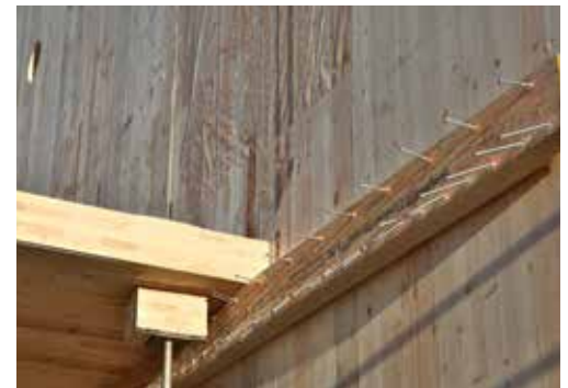
Ledger beam supporting CLT floor panels Photo Credit: Paul Alberts
