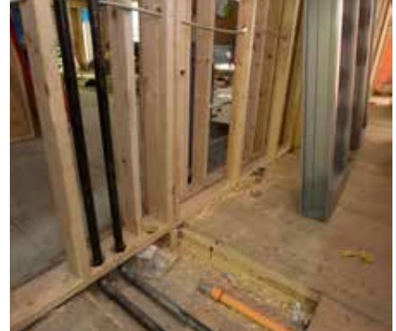
Services installed in the chases within the floor assembly Photo Credit: Paul Alberts
