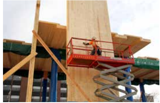
Installation of CLT wall panel against CLT lapped floor panels Photo Credit: Paul Alberts
